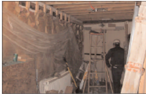
Electrical wiring continues in the backstage area.
