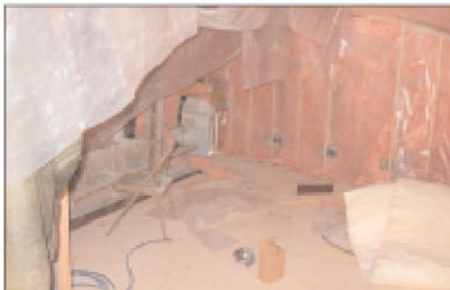
Framing of stage hands area.
