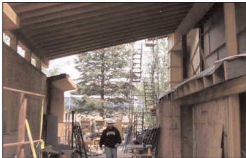
Roof over concession area has been installed.
