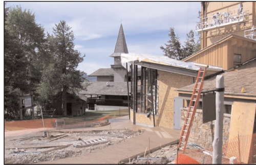
New walkway is poured outside the ticket booth area.
