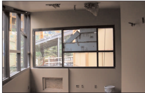
Windows in the music library have been installed.
