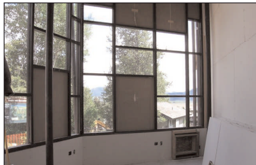
Sheetrock & windows are installed in the new ticket booth.
